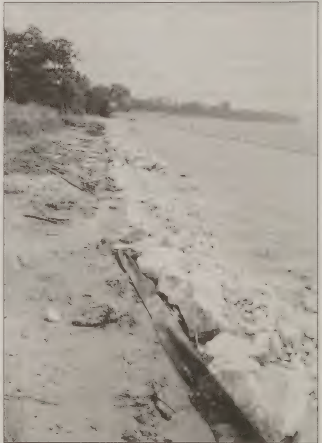
Sill and Breakwater
